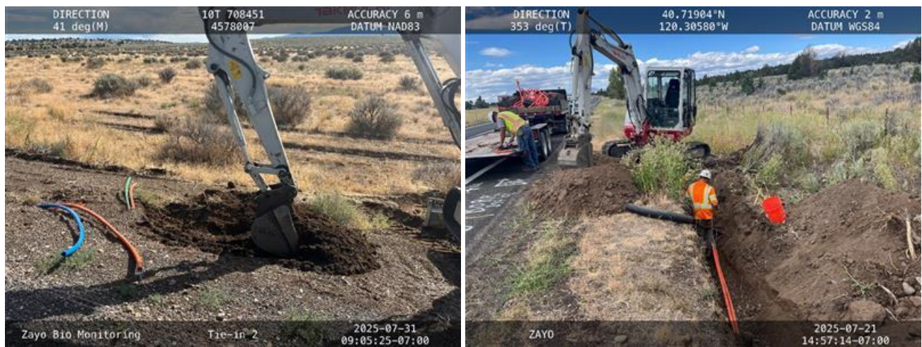
Figure 4. View of typical tie-in operations in Northern Area (Modoc County).
