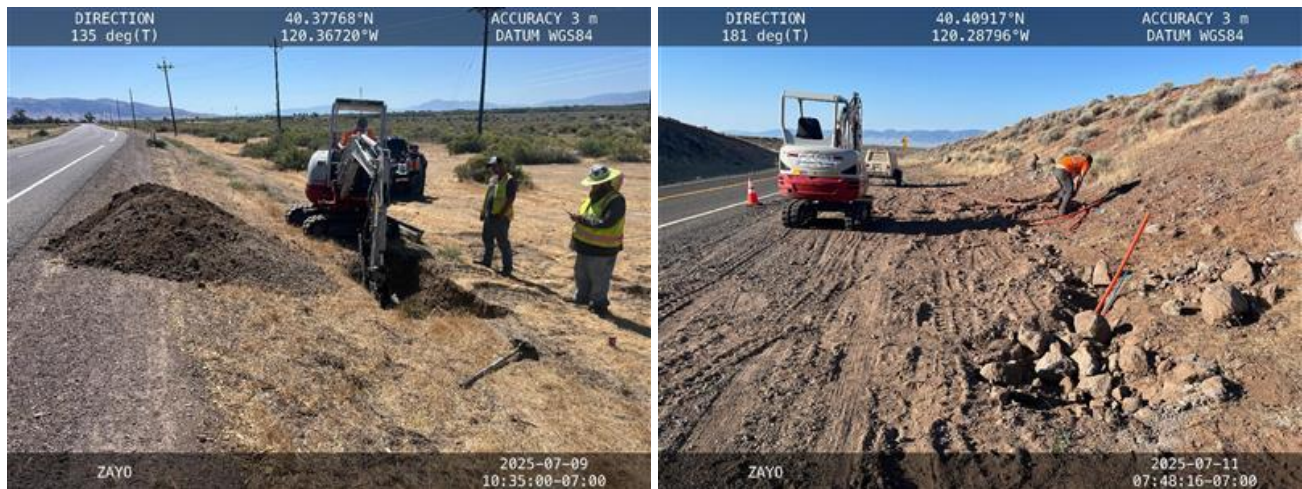
Figure 1. View of typical dig down operations in Central Area (Lassen County).
