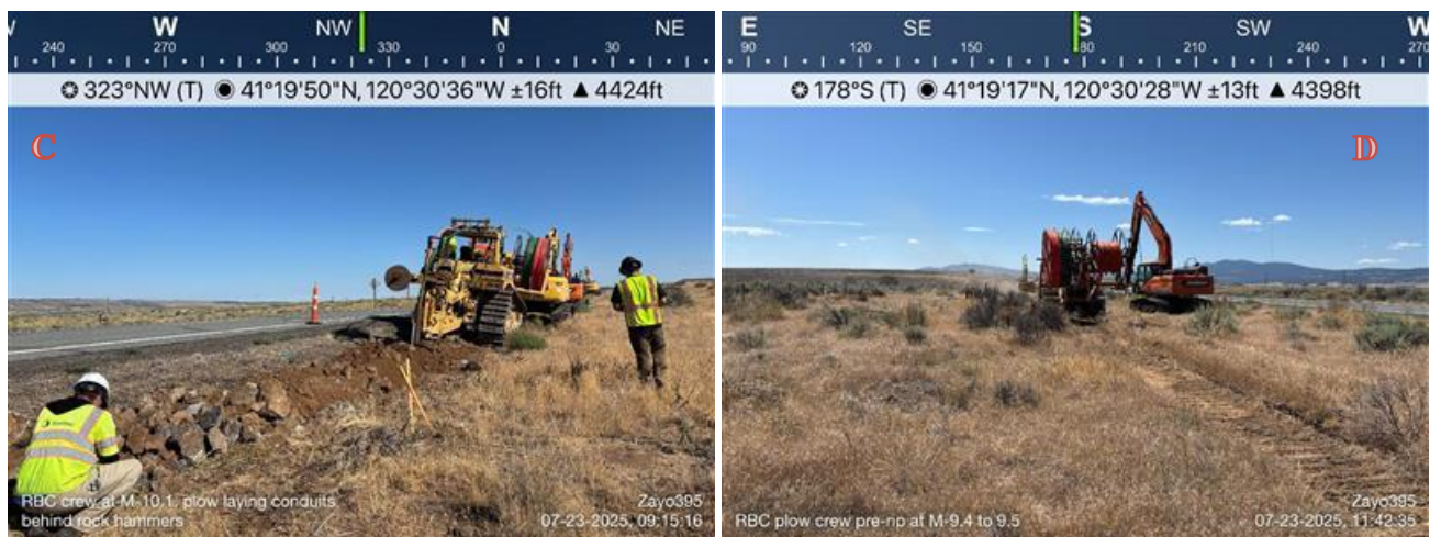
Figure 6. View of typical tie-in operations in Northern Area (Modoc County).
